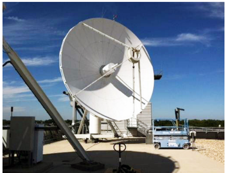
NSOF 9.1 meter antenna upgraded for GOES-R. Credit: Harris Corporation
